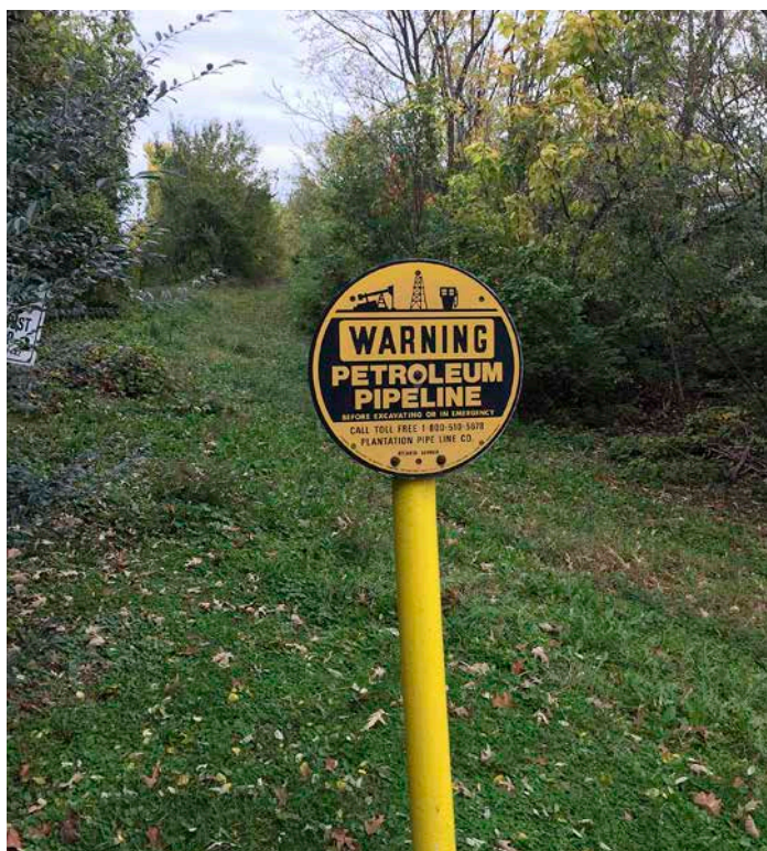
Sign indicating a buried refined-product pipeline in Alexandria, Virginia. The Plantation Pipeline runs from Gulf Coast refineries to Northern Virginia; the pipeline shown in this picture is an extension of the Plantation Pipeline that delivers jet fuel to Washington National Airport. Image credit: Ben Mandler, American Geosciences Institute.
