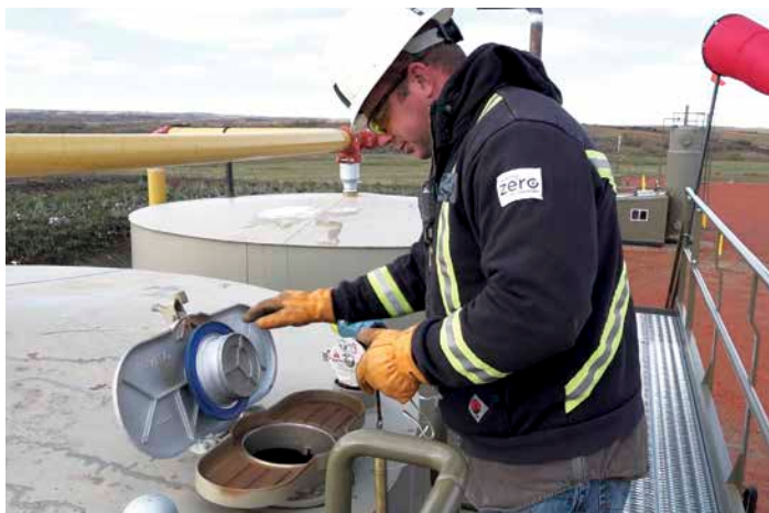
Worker gauging an oilfield tank. Tank sampling is one of the main ways in which oilfield workers may be exposed to harmful vapors. Image credit: Photo courtesy CDPH and NIOSH. 12
