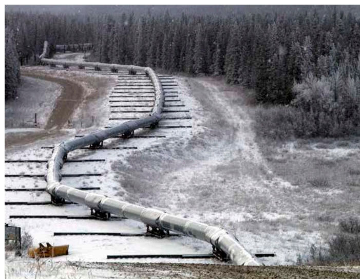
The Trans-Alaska oil pipeline is mounted on sliders where it crosses the Denali fault. During a large (magnitude 7.9) earthquake in 2002, this system allowed the pipeline to move without breaking. Image credit: Tim Dawson, U.S. Geological Survey 25
