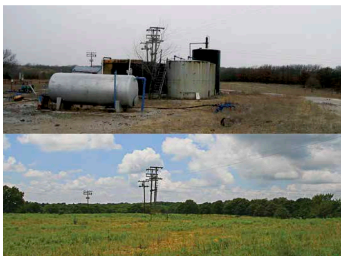
An abandoned well site in Oklahoma before (top) and after (bottom) being remediated. Image credit: Courtesy of the Oklahoma Energy Resources Board. 13
