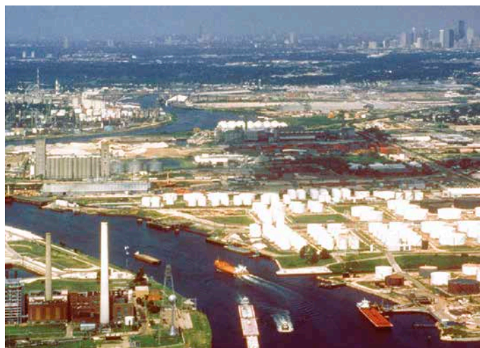
Refineries, fuel shipping terminals, and other industrial facilities along the Houston Ship Channel, 1999. The city of Galena Park is center-right. Roughly half of all U.S. refining capacity is located on the Texas and Louisiana coasts, leading to a higher risk of air pollution from refineries in this region of the Gulf Coast. Image credit: Army Corps of Engineers. 23
