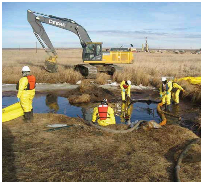
Cleanup crew at the 2015 Blacktail Creek spill, Marmon, North Dakota. This spill was caused by a leaking pipeline that was transporting produced water in the oilfield. Image credit: U.S. Environmental Protection Agency. 24
